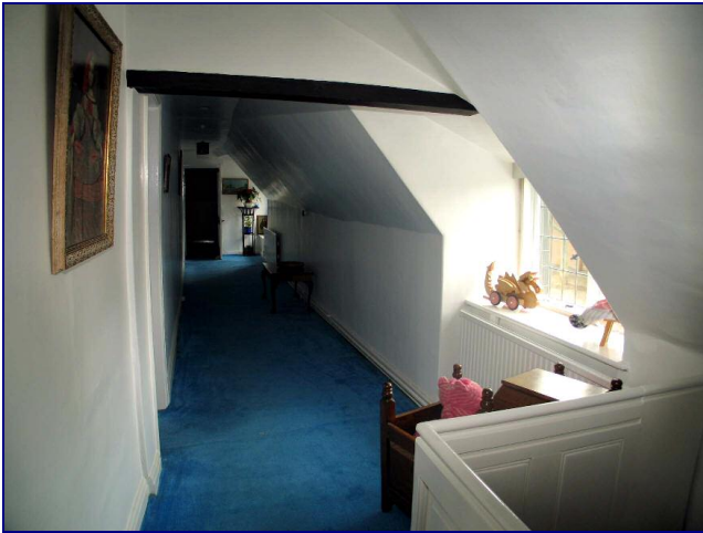
First Floor Landing
